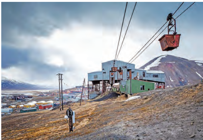
Infrastructure sits idle at the coal mine at Longyearbyen
